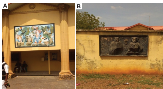
Figure 11. Indigenous art and craft sparingly expressed in the building. (A) Wall murals at the entrance. (B) Relief sculpture on the fence and sculpture in the round exhibition space. Source: Authors' fieldwork in 2019
