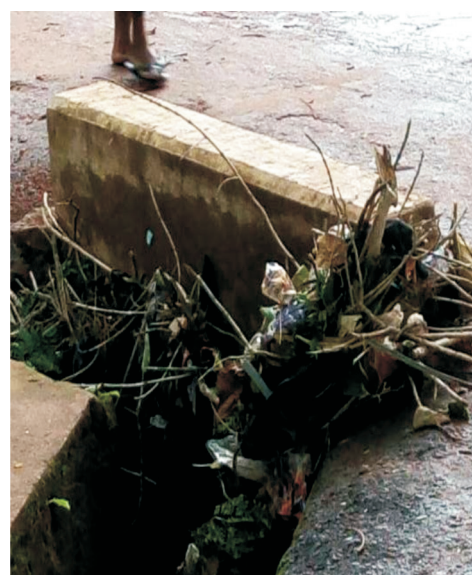
Figure 8: A culvert blocked with debris.
