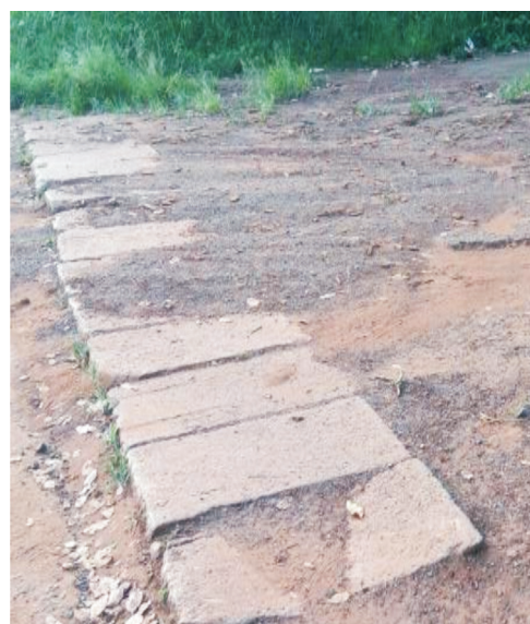
Figure 7: Silted-up culvert.
