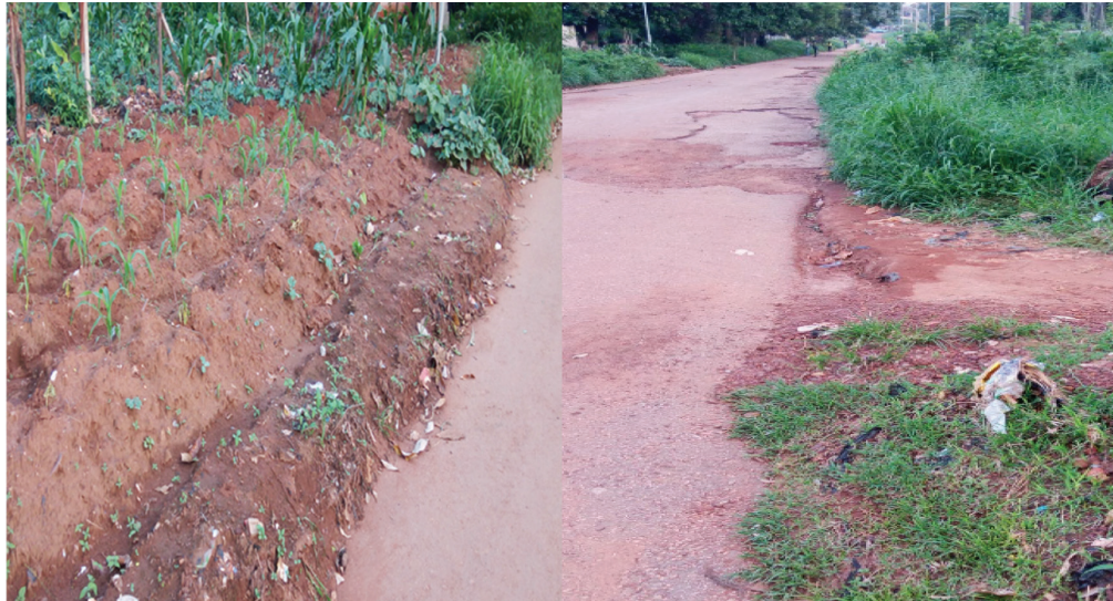
Figure 9: Ditches blocked by soil and grass verge.
