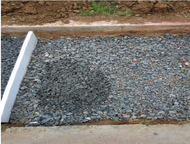
Figure 4: Filling of 20 mm aggregate for 10 cm depth.
