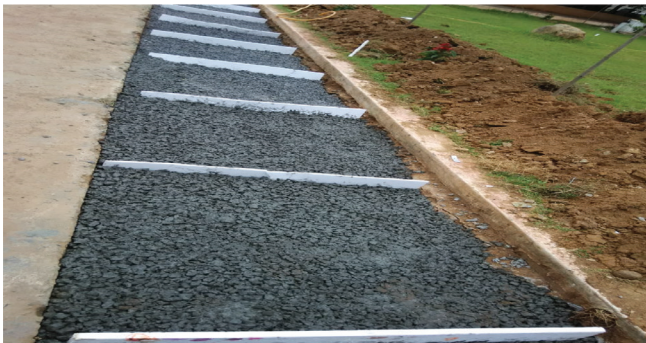
Figure 5: Pervious concrete foot path panels after laying.
