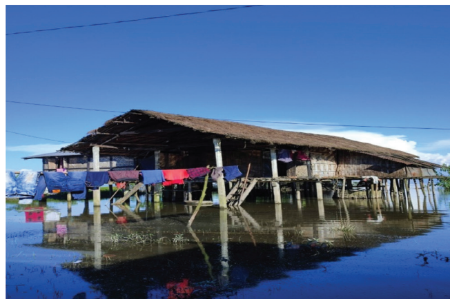
Figure 1: Flood resilient house (Chang Ghar) of the mishings.
