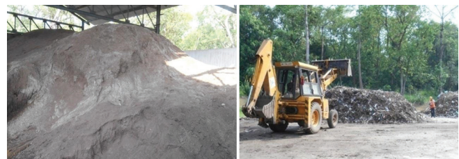
Figure 5. Composting plant at Bara Dih (windrow composting)
