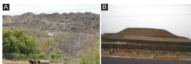
Figure 6. Disposal sites of Jamshedpur city. (A) Open dumping site at Baugun Hathu. (B) Semi-scientific landfill near XLRI, Marine Drive.
