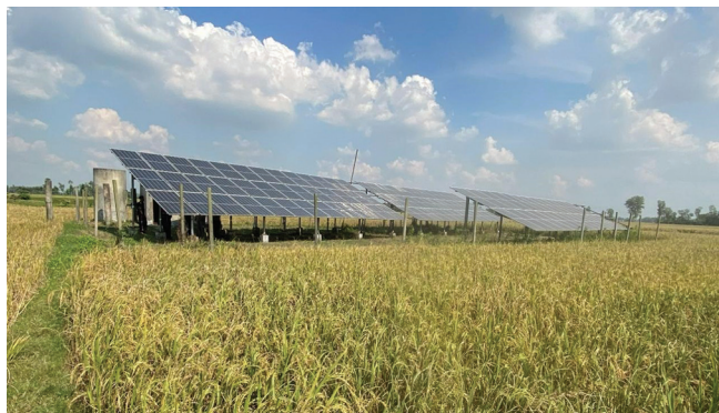
Figure 1. A solar irrigation pump well system from the study area. The solar panels supply power to the submersible pump housed within the shed located behind them. Photo by Shafiu Chowdhury.
