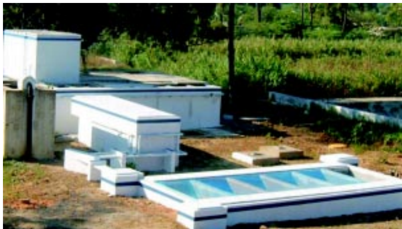
Figure 1: A view of collection tank, anaerobic baffled reactor, anaerobic filter and aerobic filters.
