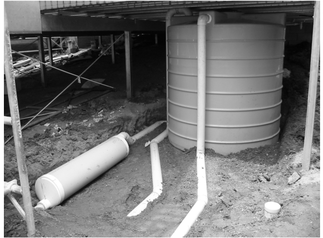
Figure 4: First flush device used in a Green Smart display home.
