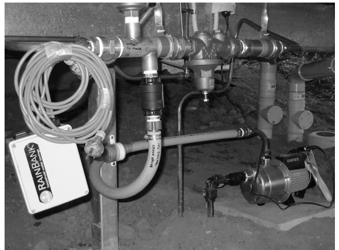
Figure 5: Pump and switching device used for uninterrupted water supply.
