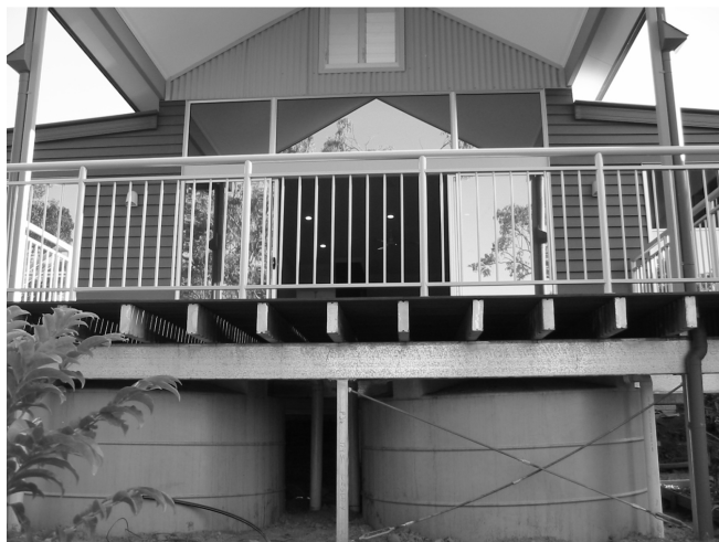
Figure 3: Water tanks placed under the elevated floor of a Green Smart display home.
