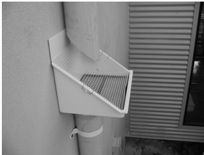
Figure 2: A rain-head installed in a Green Smart display home.
