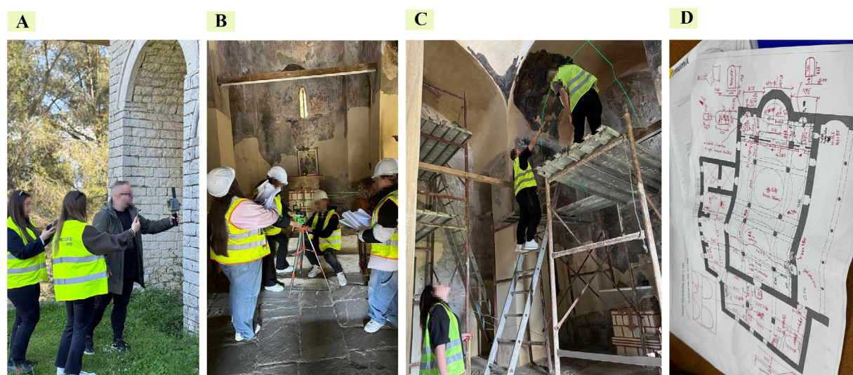
Figure 3. Fieldwork images captured during the metric survey. (A) On-site handheld scanning using an FJD Trion scanner. (B) Students' site works using a scanner-meter to measure the interior geometric data of the church. (C) On-site leveling measurements by students. (D) Dimensions sketches were made on-site during the metric survey process.
