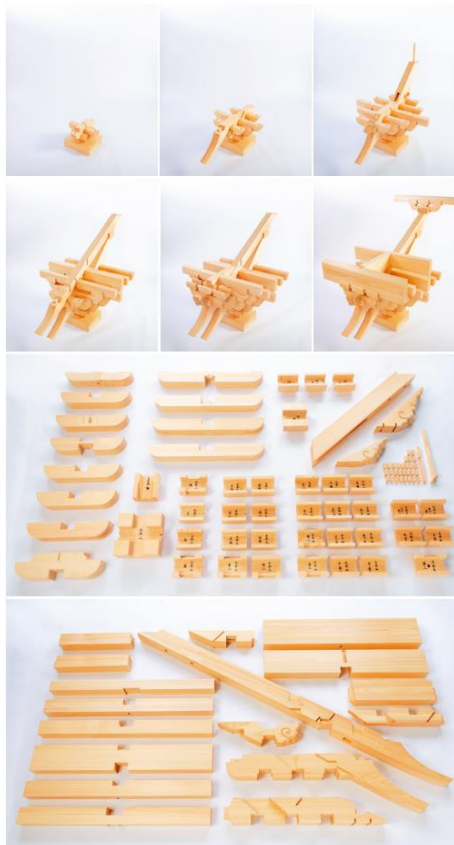
Figure 5. Decomposition model of the bracket sets under the eaves of the Shariden Hall of Engakuji Temple in Kamakura. Source: Produced/collected by Takenaka Carpentry Tools Museum
