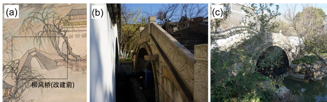
Figure 1. Liufeng Bridge. (a) Detail of Figure 9. (b, c) Pictures photographed by the author.
