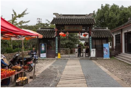
Figure 3. Entrance gate to Mingyuewan Historic Village, located in the south of Xishan Island in Lake Tai. The settlement is designated as a historical and cultural village, and a national agricultural tourism demonstration pilot project. Source: Photo by the author, 2017
