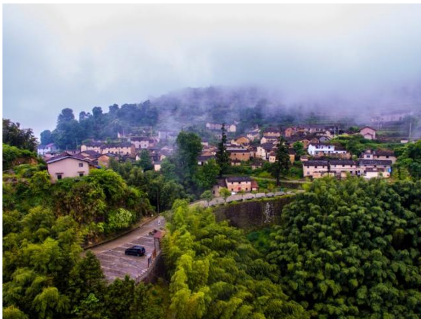
Figure 2. Pingtian Village after 2 years of planning and reconstruction. Source: Yunshang Pingtian Guesthouse
