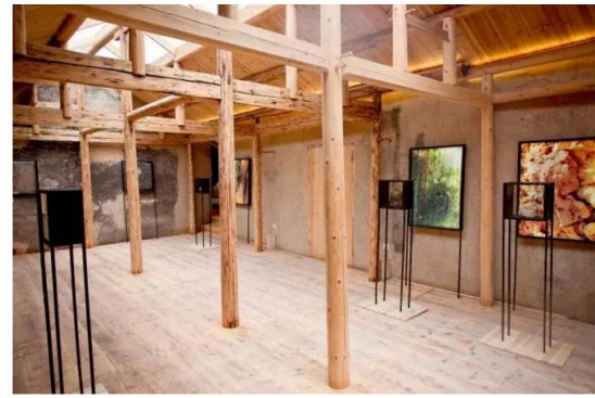
Figure 13. Interior of Pingtian Agriculture Hall after the renovation. Source: Photo provided by DnA Architects
