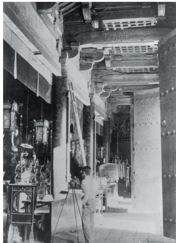
Liang Sicheng surveying and mapping the main hall of the Foguang Temple in Mount Wutai, Wutai County, Xinzhou, Shanxi Province, China (1937)
