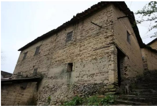
Figure 10. Pingtian Agriculture Hall before the renovation. Source: Photo by Junjie Li
