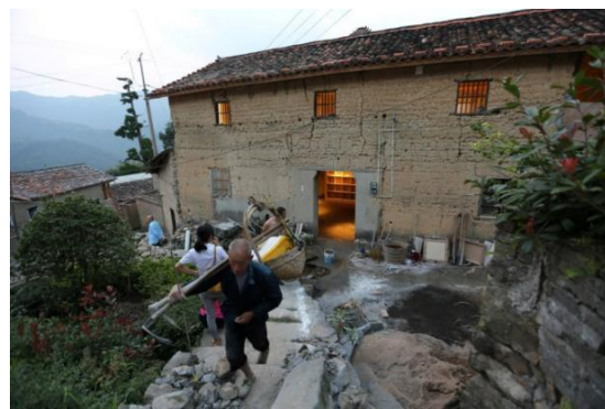
Figure 14. Papa's Hostel after the renovation. Source: Photo provided by 3andwich Design
