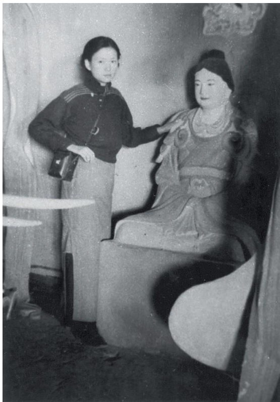
Lin Huiyin at the main hall of the Foguang Temple in Mount Wutai, Wutai County, Xinzhou, Shanxi Province, China (1937)
