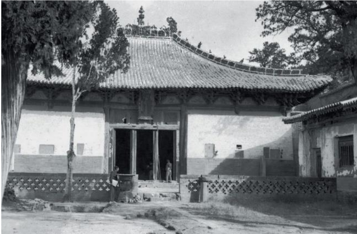
Liang Sicheng surveying and mapping the main hall of the upper temple in the Guangsheng Temple, Zhaocheng, Hongtong County, Shanxi Province, China (1936)
