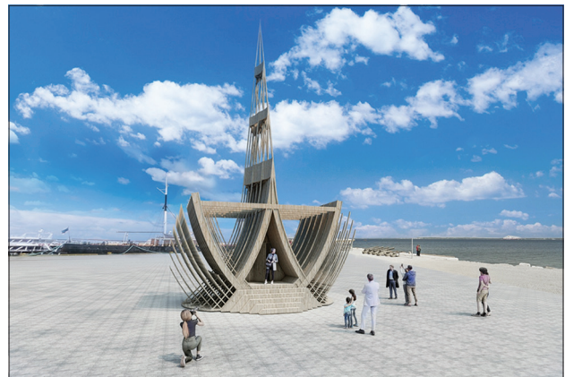
Figure 9. Microbial fuel cells toilet structure made from recycled wood, inspired by ship hulls at Seaplane Harbour. Source: Concept for the Estonian Maritime Museum, Tallinn, rendering by Anna Vershinina; courtesy of Anna Vershinina, 2023.
