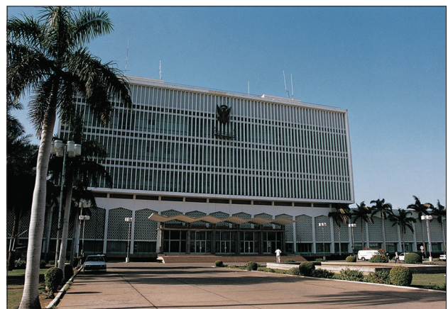
Figure 20. The main volume of the Friendship Hall. Source: Shanghai Institute of Architecture Design and Research.
