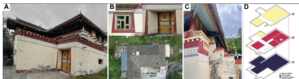
Figure 8. Illustration of typical dwelling features of partially reconstructed A dwellings. (A) Appearance; (B) construction; (C) structure; (D) floor plan showing functional zones. Source: Photos and drawing by the authors
