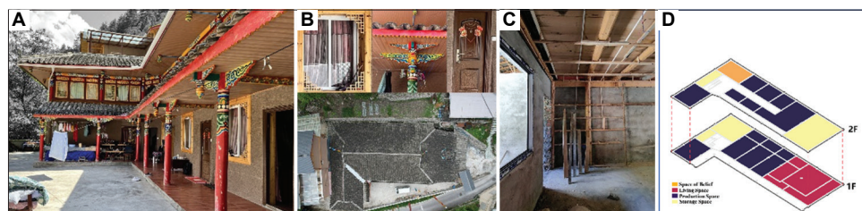
Figure 9. Illustration of typical dwelling features of partially reconstructed B dwellings. (A) Appearance; (B) construction; (C) structure; (D) floor plan showing functional zones. Source: Photos and drawing by the author
