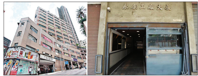
Figure 3. The withdrawal case of Cheung Hing Industrial Building and the partly renewed case of Wing Hong industrial building. Source: https://hk.on.cc/hk/news/
