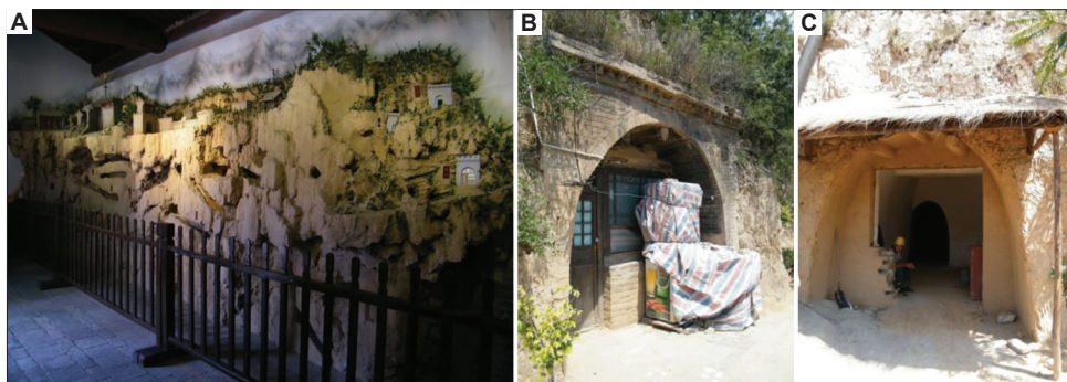
Figure 6. Zhangbi village, Jiexiu City, Shanxi province, 2018. (A) A diorama illustrating the structure of the hill, with the city built on top of the network of underground tunnels. (B) An old yaodong, along the slope of the hill facing the valley, used as a tourist shop. (C) Renovation of a yaodong connected directly to the tunnel network. Source: Photos by Laura Genovese
