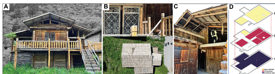
Figure 7. Illustration of typical dwelling features of traditional dwellings. (A) Appearance; (B) construction; (C) structure; (D) floor plan showing functional zones. Source: Photos and drawing by the authors
