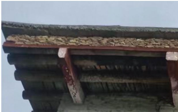
Figure 27. Roof structure. Source: Photo by the authors
