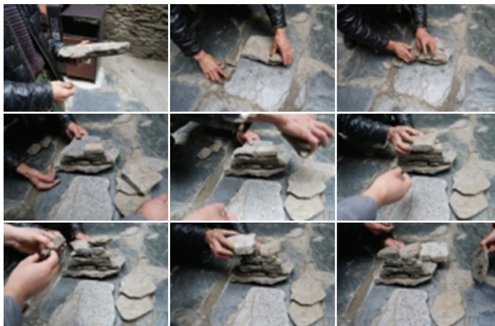
Figure 23. Traditional Diaolou construction skills. Source: Photos by the authors
