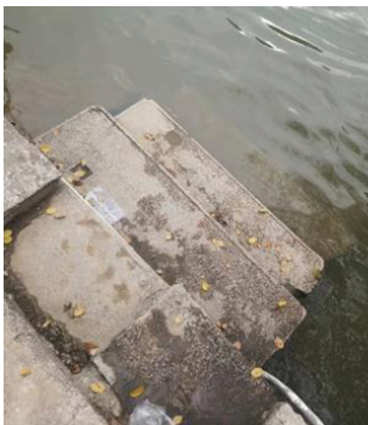
Figure 9. Damaged stone tablets commemorating nominees who passed the highest-level Imperial Examinations. Source: Photo by the authors
