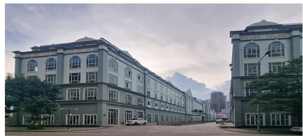
Figure 7. Peri-urban shophouses in Phnom Penh, Cambodia Source: Photo by the author (2024).
