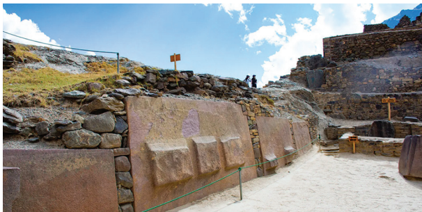
Figure 4. Cuts in the bedrock for the formation of platforms. Photographic and sectional evidence illustrating rock-cutting techniques and surface-finish variations used in the construction-technique comparison (Table 3) Source: Photo taken by the authors (2025)
