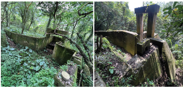
Figure 10. Remains of the forebay tanks of the two power plants responsible for supplying the Hualien Port. Left: Shapodang II. Right: Shapodang I.
