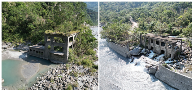
Figure 5. Once a pinnacle of the Japanese Hydropower Industry, the remains of the old Tongmén powerhouse. Left: The tall generator hall in the foreground of the powerhouse. Right: The remaining ruins of the second Qingshui powerhouse background structure, built initially behind the powerhouse turbine and generator hall, still stand along the Mugua River. Both power plants faced the same fate: being entirely flooded, silted up, and subjected to severe landslides.
