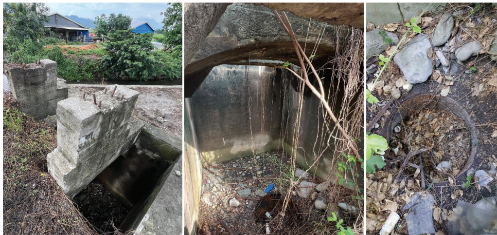
Figure 3. Pictures from the excavation process. Left: Remaining hydraulic structures of the turbine pit and generator platform of the Guanshan hydropower plant. Middle: The open-flume vertical-axis Francis turbine installed in the powerhouse. Right: Only the tailrace draft tube at the bottom of the turbine pit remains visible.
