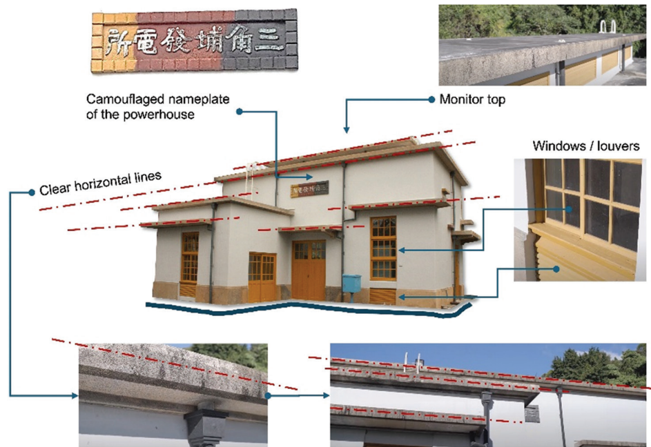
Figure 4. Elements of the Sanjiaopu hydropower plant, built at the bottom of the Caoshan waterway. Sanjiaopu is the only hydropower plant in Taiwan that utilizes tap water from Artesian wells, and it is also the only power plant designed after the water treatment process, demonstrating the cleanliness of hydropower technology.
