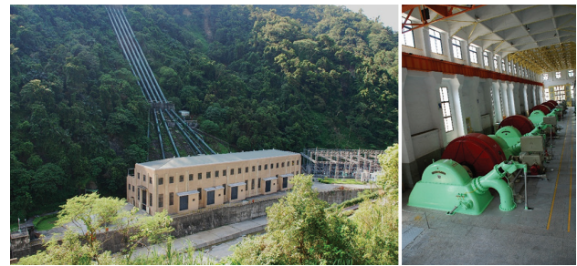
Figure 11. Daguan I, a powerhouse. Left: The penstock. Right: Turbine hall.
