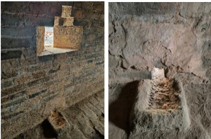
Figure 1. Wall thickness, roof drainage, and structural layering. Source: Photos by the authors
